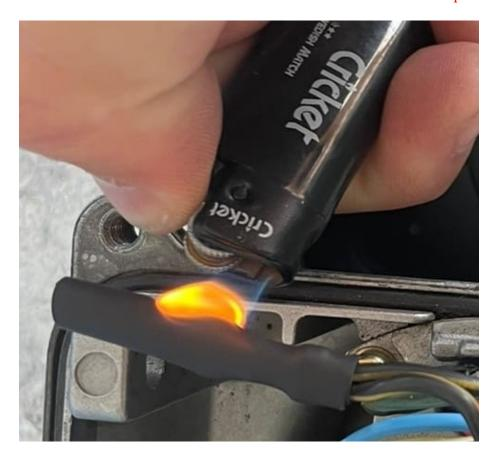
\* Use 5mm (0.2 in) heatshrink tube to insulate wire with ring terminal.
